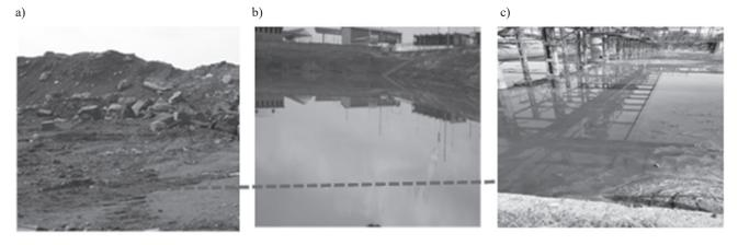
Fig. 2. Formation of residual water at the storage sites of phosphorus-containing waste. a) Phosphorus-containing slags; b) Collection of stormwater and residual water in lowlands; c) Collection of residual water in concreted reservoirs.
